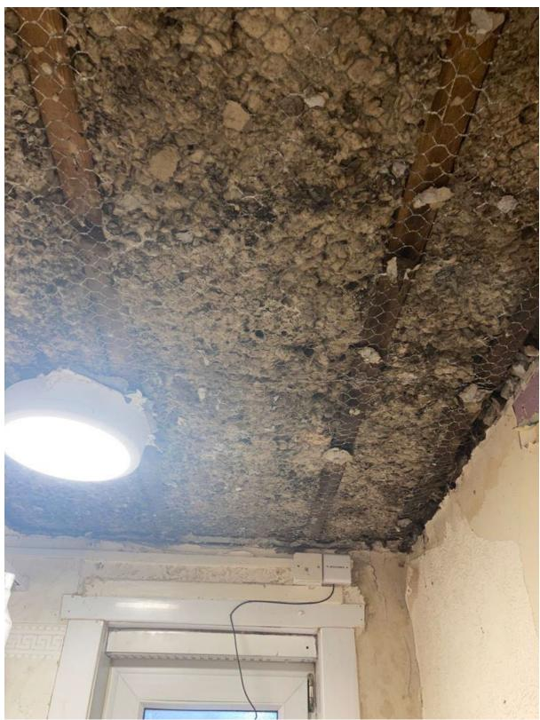
**Note**: This client's bathroom ceiling fell down over 4 years ago, due to damp. The local authority has failed to repair this, leaving the tenant to live with this ceiling, which is now infested with insects which often fall onto the client when using the room.
