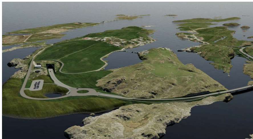
The 25.4-kilometre Rogfast tunnel in Norway. Image courtesy of COWI
