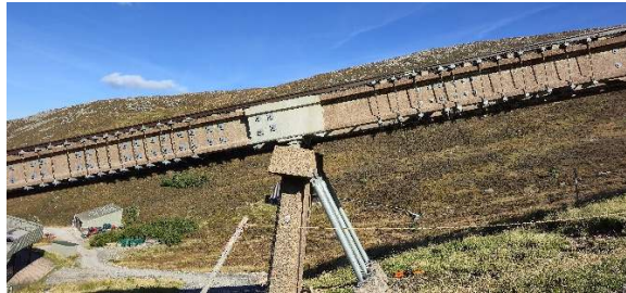
Steel struts installed on the uphill side to limit pillar rotation
