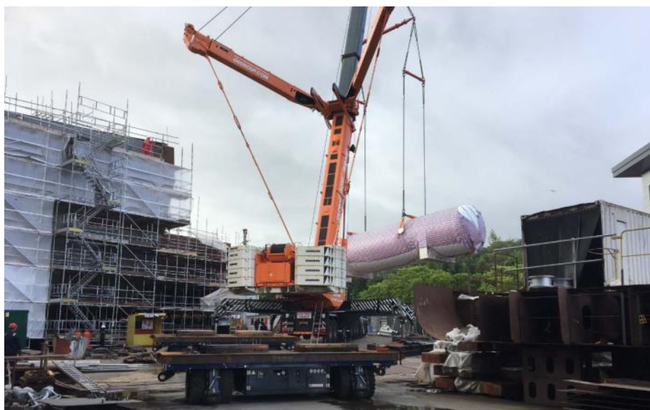
figure 3-27 801 lifting the tank on to the bow of deck 3
