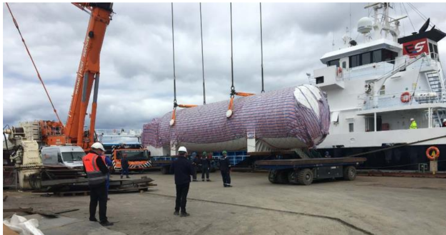
figure 3-26 lifting the tank on to the slipway upon delivery
