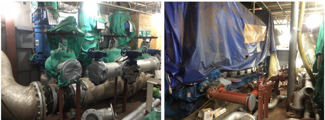
figure 3-34 engine room outfitting
