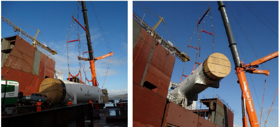
figure 3-29 tank being hoisted on deck 3 of hull 802
