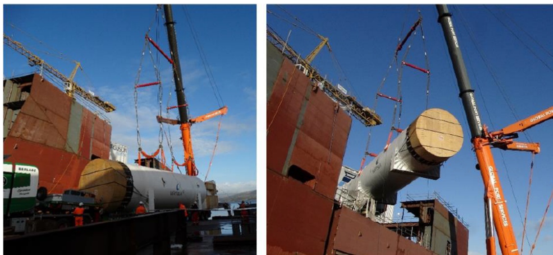
figure 3-29 tank being hoisted on deck 3 of hull 802
