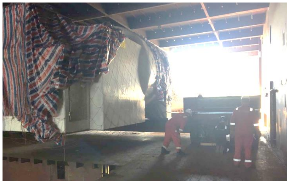
figure 3-28 positioning tank over opening at deck 3 showing cradle and removal of SPMT's
