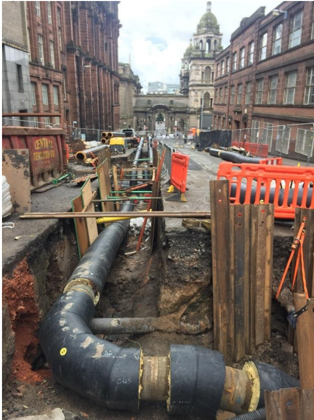
District Heating Pipework Installation underway in John Street, Glasgow.
