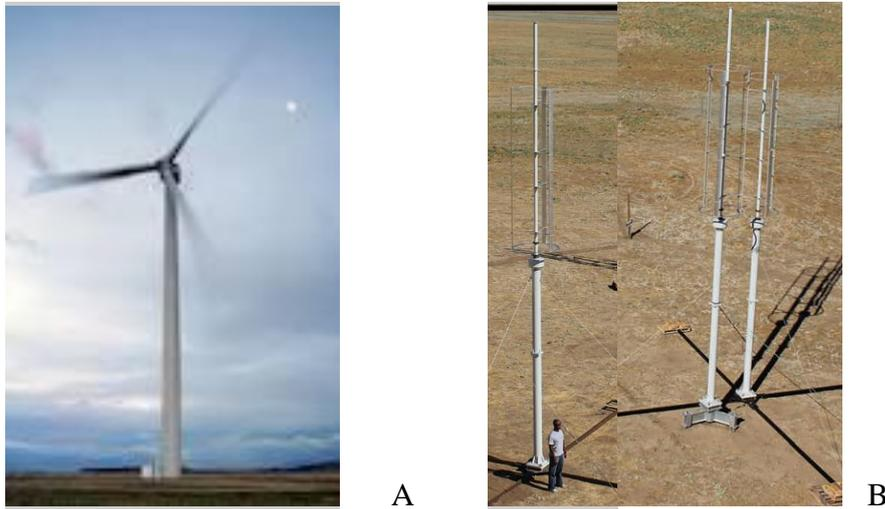
*Figure 1. Typical horizontal axis propeller-style wind turbine (A) and the type of vertical axis wind turbines used by Professor Dabiri, one of many commercial designs (B).*
